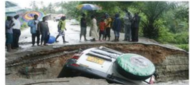
Flooding in Dar es Salaam on 26/10/2019
